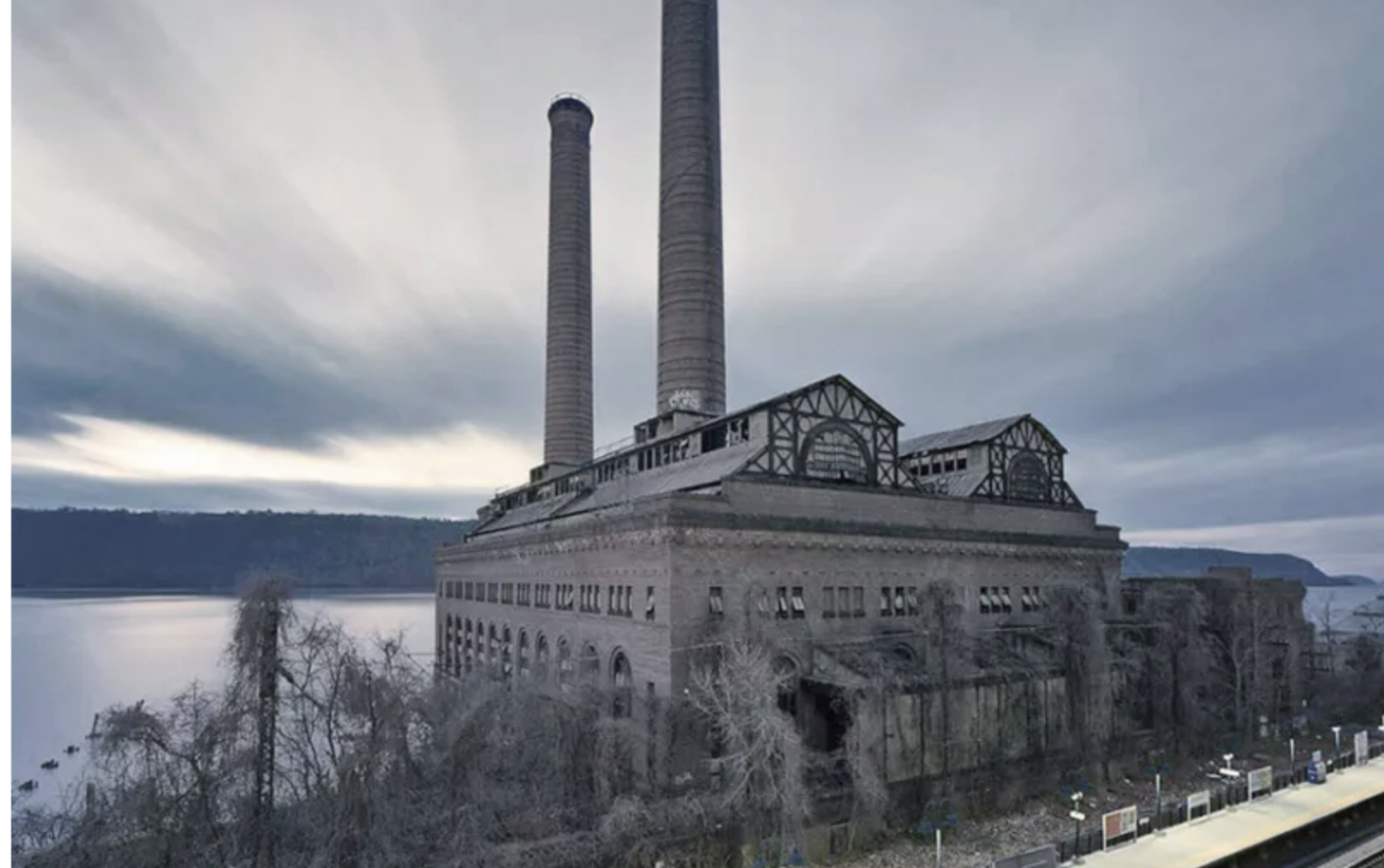
Railroad Power Station, Glenwood NY
