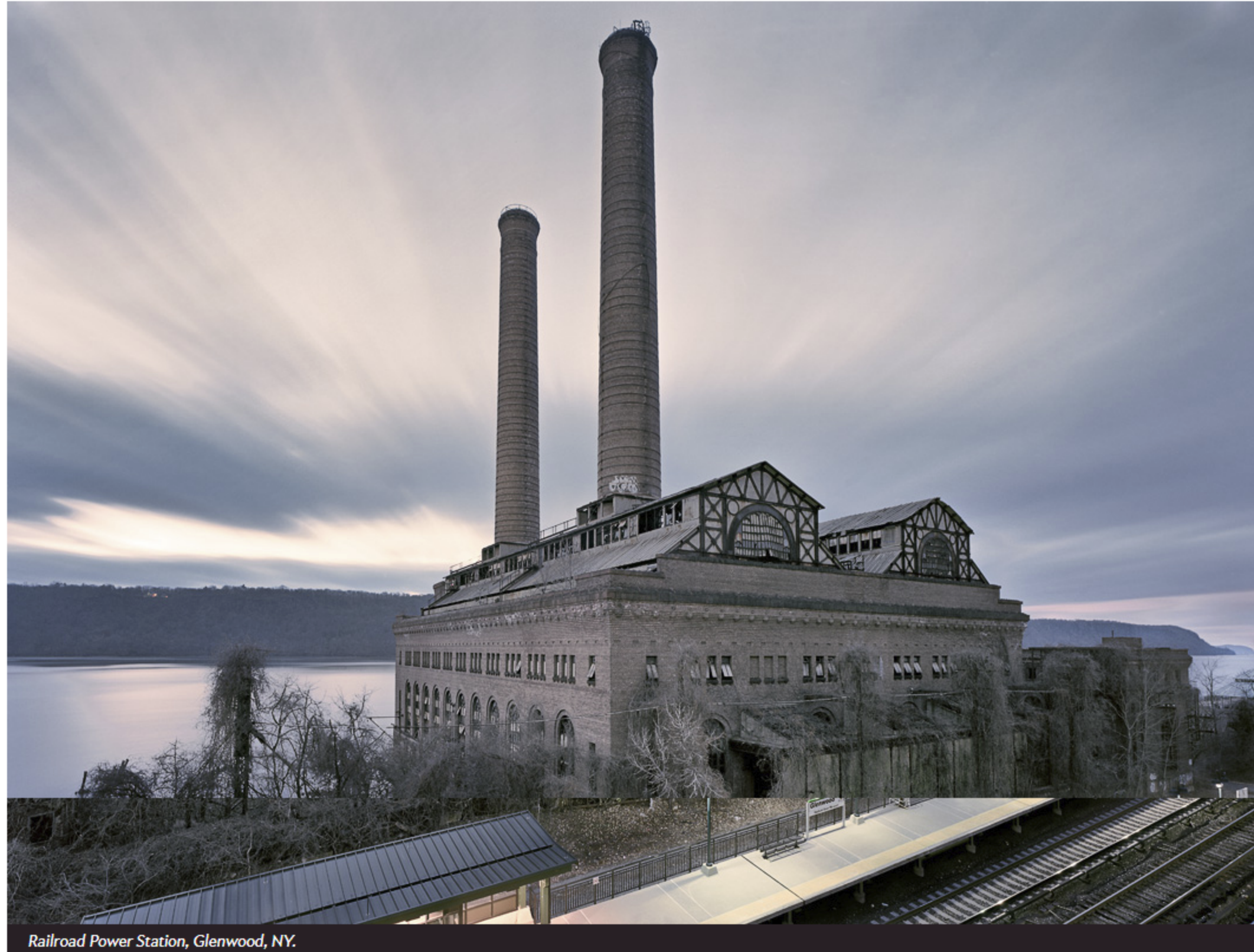
Railroad Power Station, Glenwood, NY.
