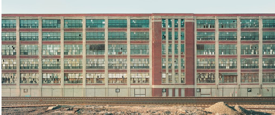
Studebaker Plant, South Bend, Indiana
